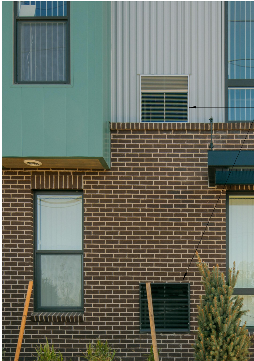
MECHANICAL LOUVER EXAMPLE: THROUGH-WALL LOUVER SYSTEM FINISH TO MATCH ADJACENT CLADDING MATERIAL.
