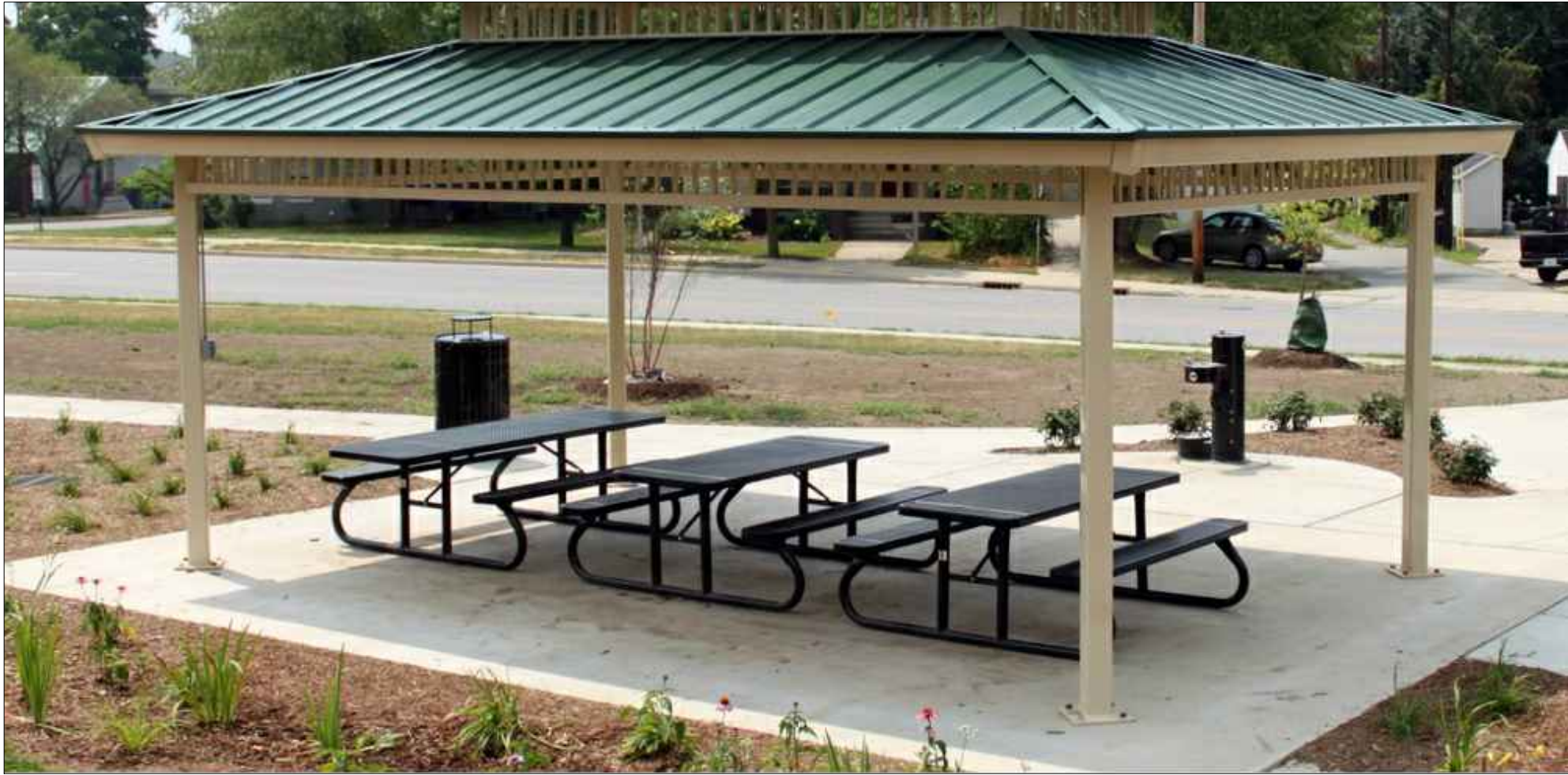
3 SHADE STRUCTURE SCALE: NTS DIMENSIONS: 13' X 14' POST TO POST
