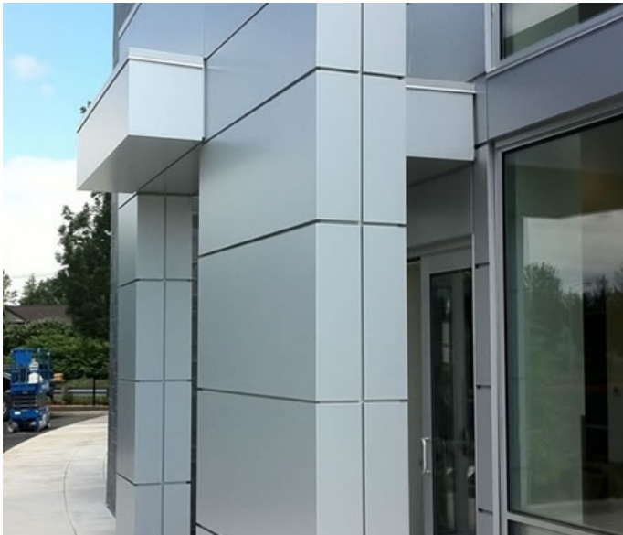
EPS-1 ALUMINUM WALL SYSTEM MANUFACTURER : CITADEL - ENVELOPE 2000 RAINSCREEN COLOR : CLEAR SATIN ANODIZED
