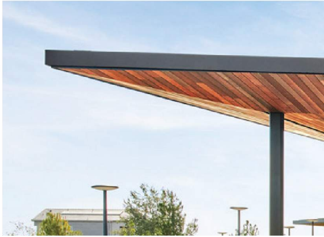
A ROOF FASCIA, T&G FACETING, AND STEEL COLUMNS
