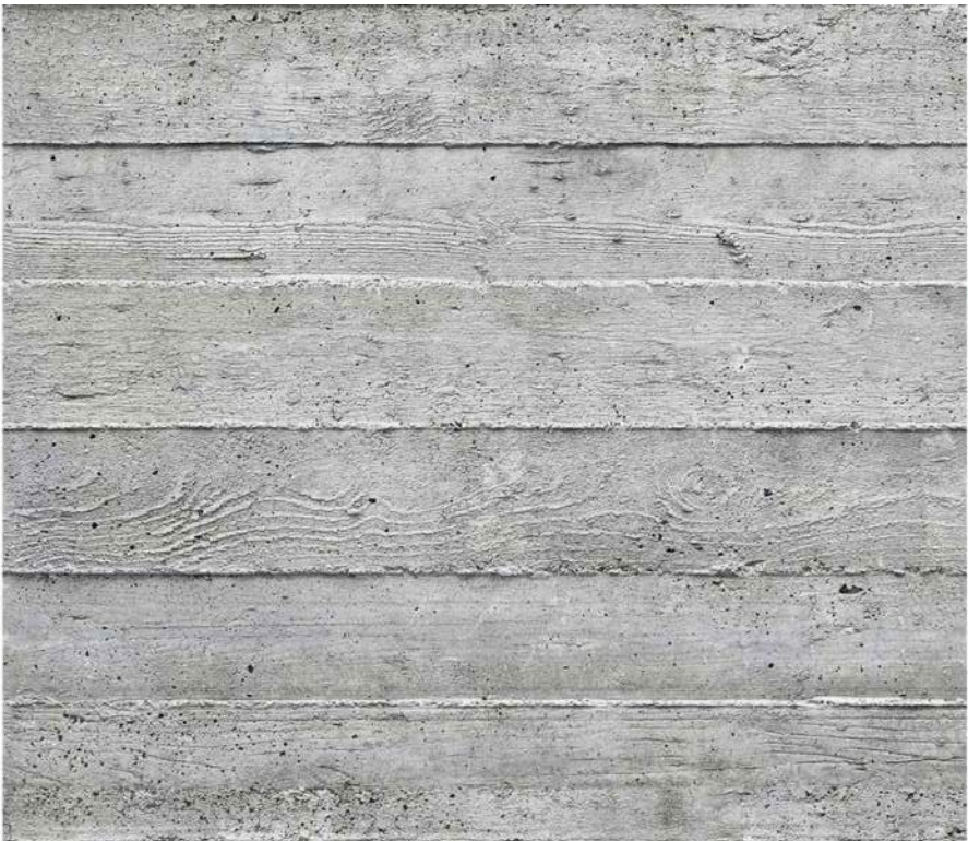
B BOARD FORM CONCRETE OR SIMILAR - BOARD SPACING AND REVEAL MAY VARY
