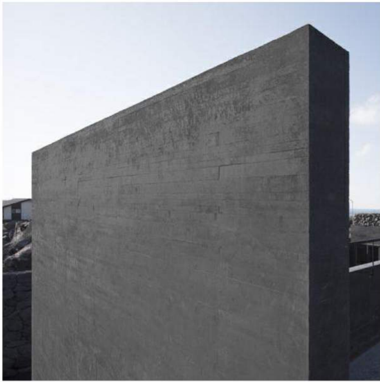
B CAST-IN-PLACE CONCRETE WALL AND SEATING HEARTH W/ INTEGRAL COLOR AND TEXTURE/AGGREGATE
