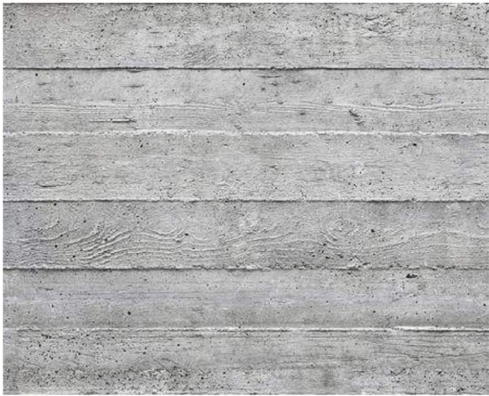
C CAST-IN PLACE BOARD FORMED CONCRETE
