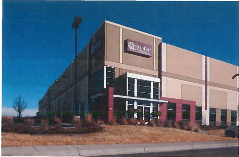
7A. Entrances differentiated from warehouse building with articulated features, interlocking forms and accent colors
