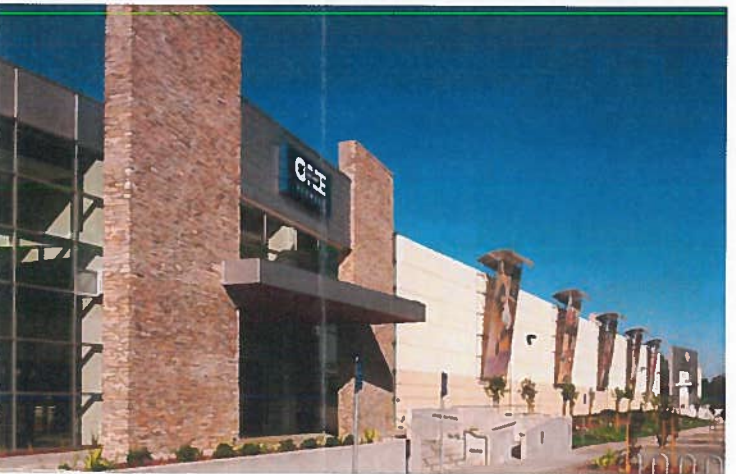
7F. Main entrance emphasized with canopy and fenestration features and textured finishes; Large adjacent warehouse facade broken up with screenwall features
