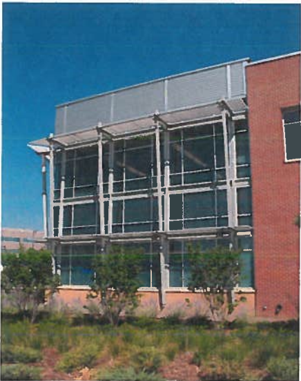
5B. Functional sun-shade devices integrated with window design
