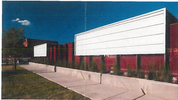
6B. Overlapping of roof and screening forms and utilizing contrasting color integrated with landscaping
