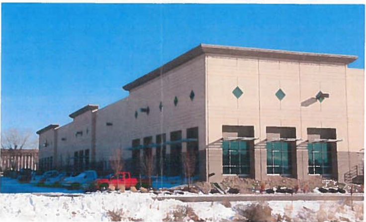
7B. Use of functional shading devices at fenestration; and long facades broken up with plane changes and variations in wall
