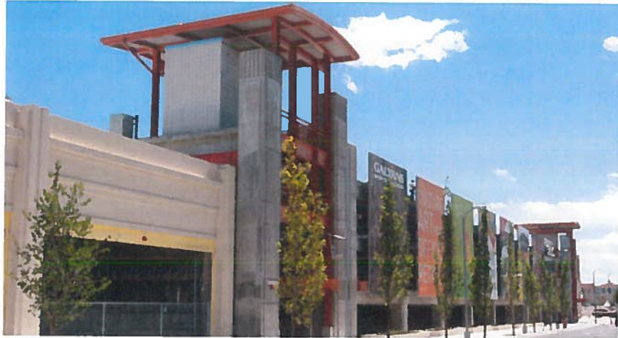
6A. Architectural screening devices shield parked vehicles and double as signage
