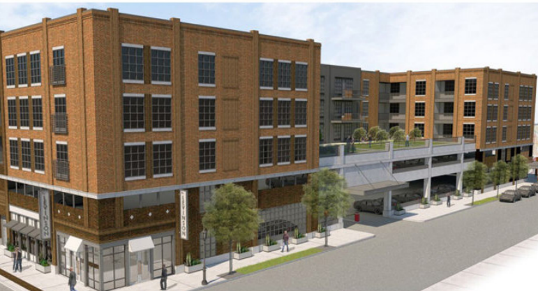
a good example of wrapping a parking garage with building massing to disguise and limit the visibility of the parking area from adjoining streets.
