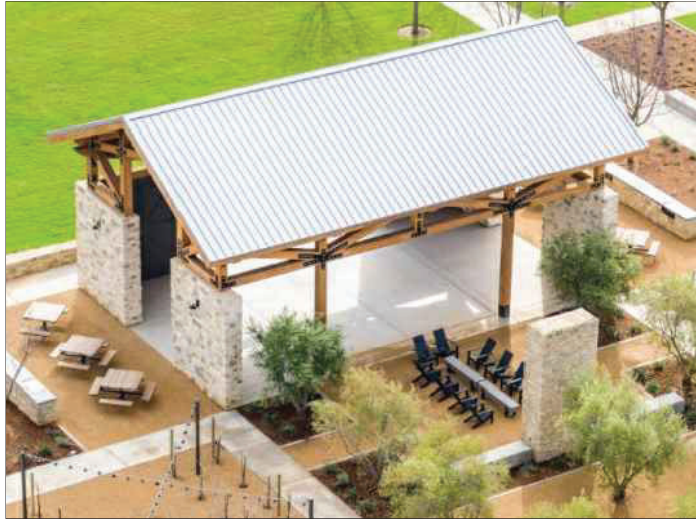
1 SHADE STRUCTURE NTS (Images for reference only) DIMENSIONS: 14' X 20' MATERIALS: VENEER: STONE BEAMS: WOOD ROOF: STEEL
