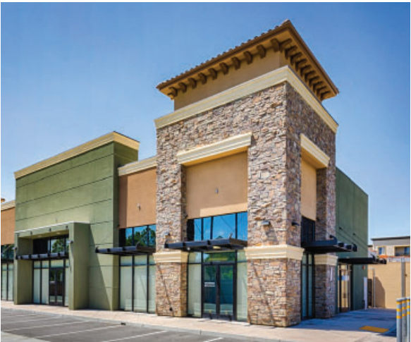
Vertical building elements define entrances and make the building identifiable
