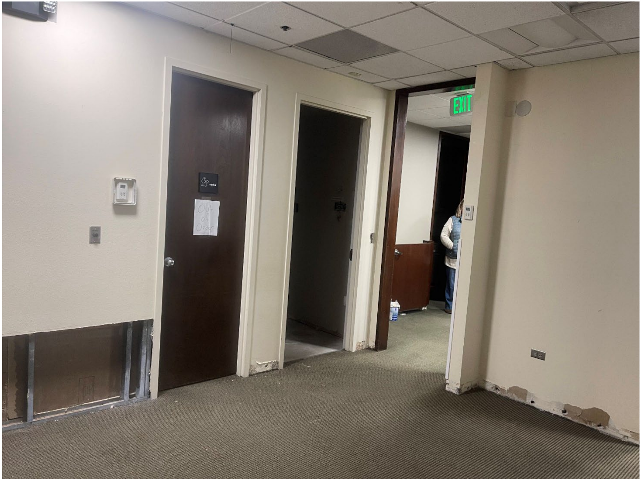
Figure 2. Taken from the basement, this photo show damage to the floors, walls, and ceilings. This basement space is connected to the 1 st floor bank space and was at one time used for the vault and storage.
