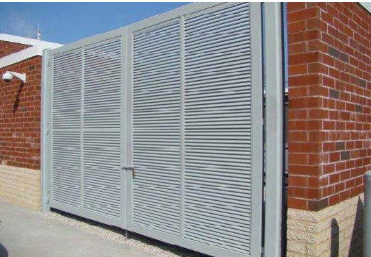
Figure 4.26: Outdoor service area screens shall be masonry or an approved alternate.
