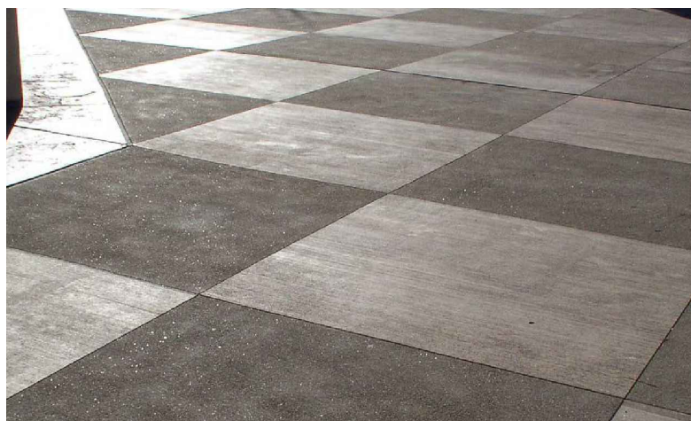
Decorative Paving (directional broom finish)
